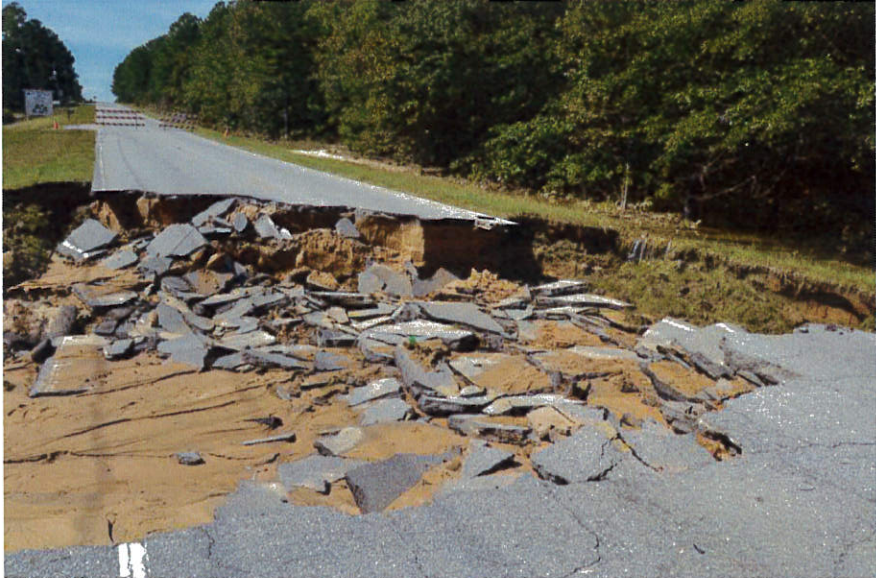
Crossline pipe failure
